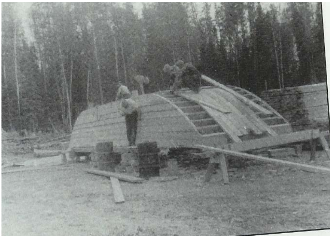
One of Patricia's Scows under construction.
