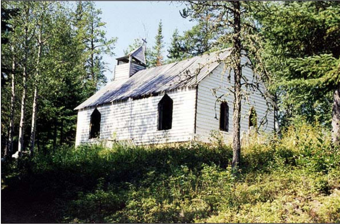
St. John's Parish Church before restoration.
